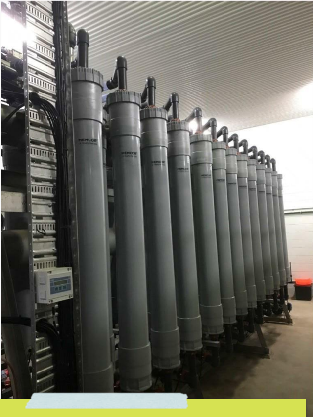
Membrane replacement works at the Mossman and Whyanbeel WTPs
